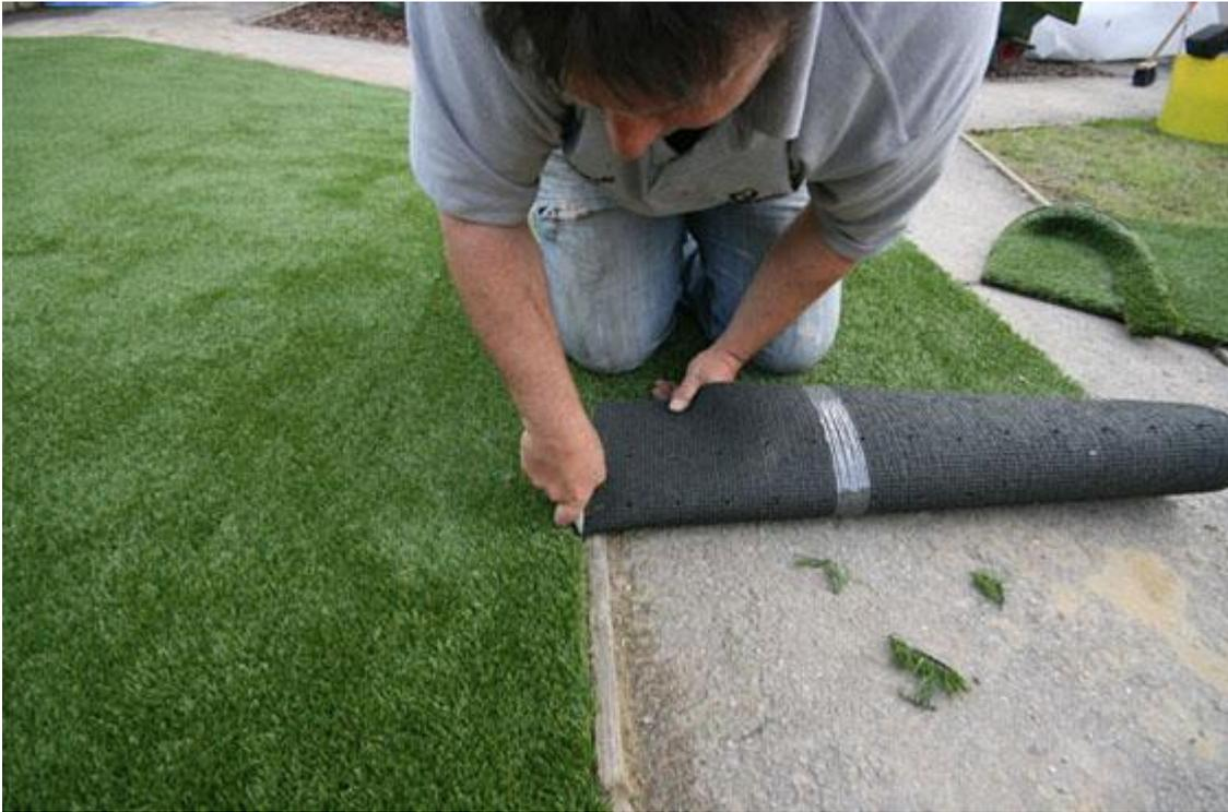
**Once the glue has bonded you can trim the edges, again making sure you are using a sharp Stanley knife.**
