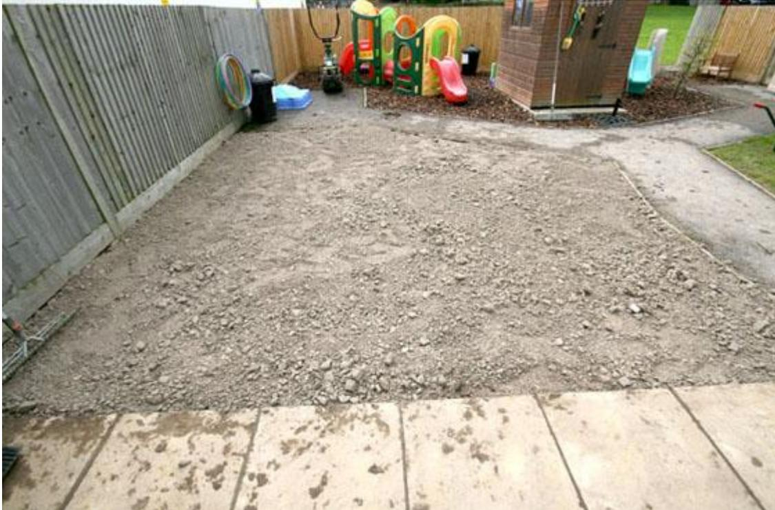
**Make sure the Type 1 is evenly spread, smooth off any humps with a rake. Compact the Type 1 with a wacker plate and blind off with a thin layer of sharp sand.**
