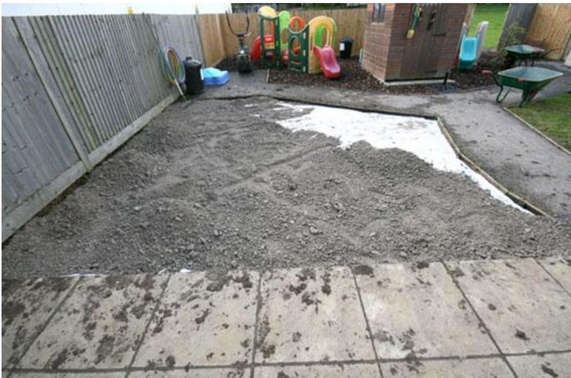
**Install the first layer of geotextile weed membrane on top of the soil. This will prevent the sub base sinking in to the mud. Fill the area with Type 1, sometimes known as**
