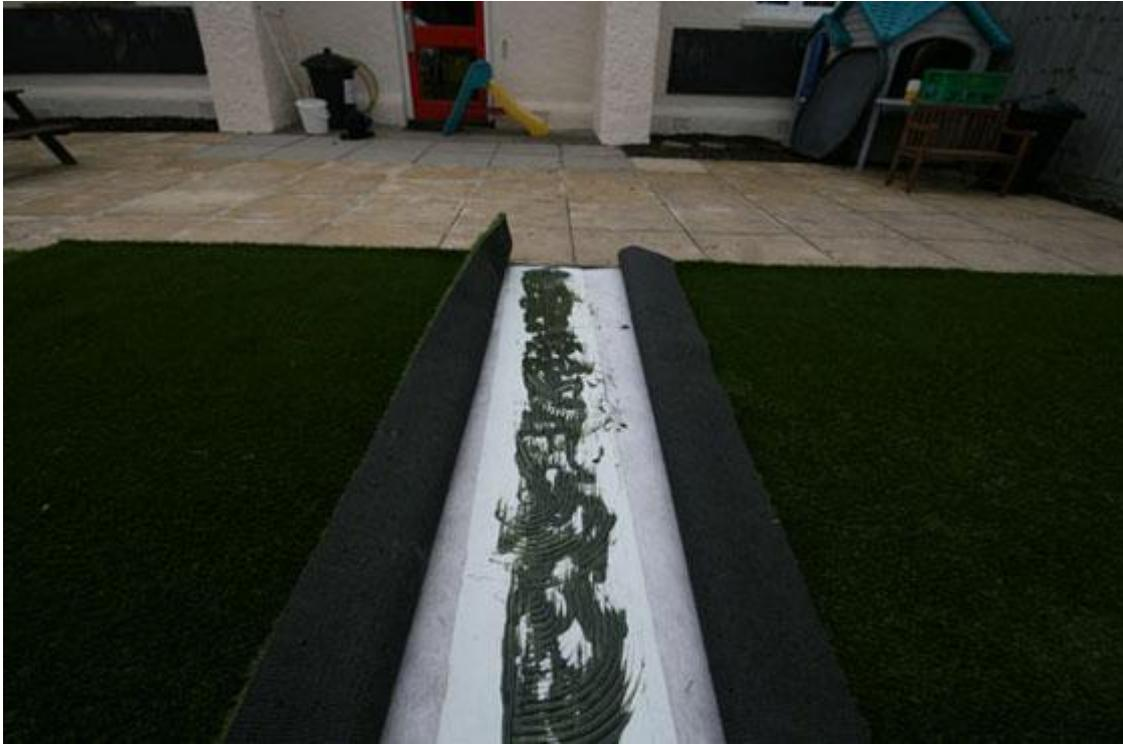
**Once you are happy the two pieces of grass are butted up exactly, fold both pieces back and lay the joining tape evenly between them. Apply the glue to the joining tape and spread with a toothed trowel. Carefully fold both pieces back and apply pressure to the join. Make sure the glue is not too thick or it will push through the join or the drainage holes.**
