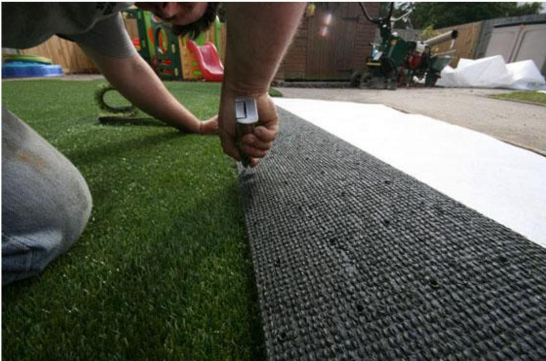
**When joining two pieces of grass together, cut evenly down the stitch lines on each piece of grass. Butt the two pieces together and check the join. It is quite possible there is still some trimming to be done.**
