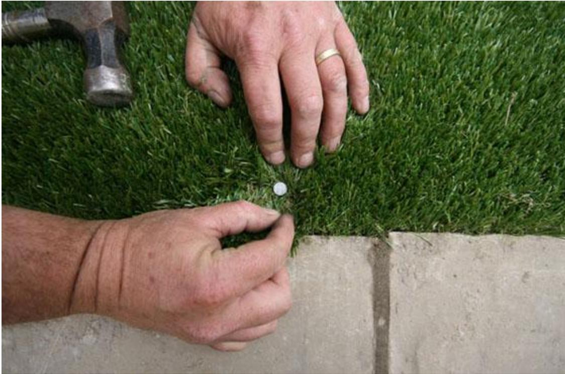
**Hold the pile open and tap the nail in so the head of the nail is just touching the latex backing of the turf. Once in position, release the pile so it covers the nail.**
