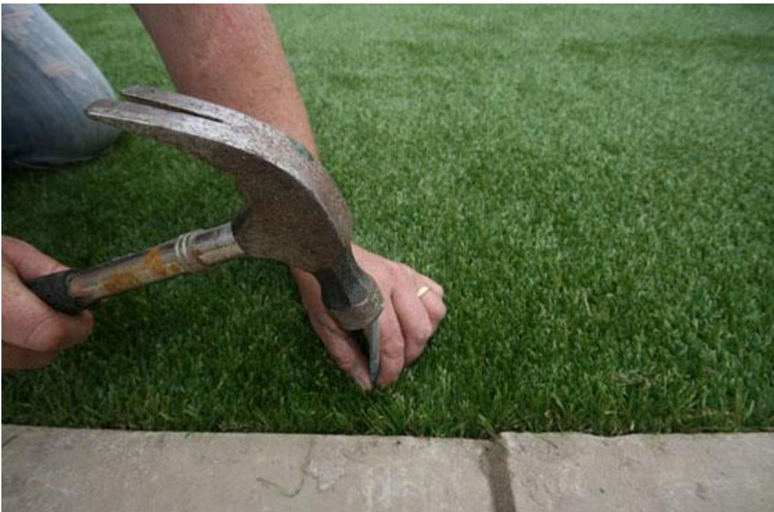
**Using 6 inch galvanized nails, pin the turf every 6 – 12 inches around the edge.**
