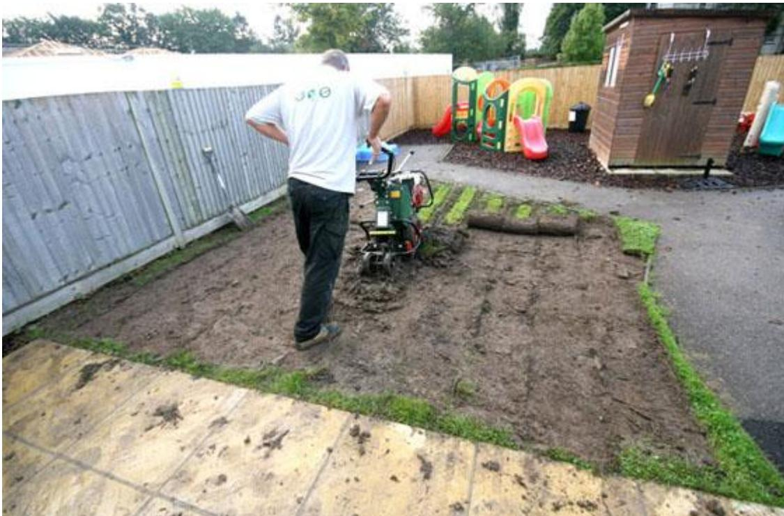
**Using a turf cutter, remove the turf to a depth of 2 – 3 inches. Free draining lawns will require a 2 inch base; poor draining lawns will require a 3 inch base.**
