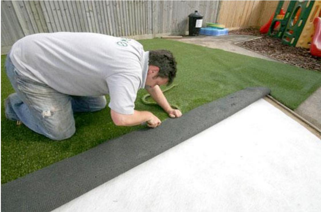
**Lay the artificial grass out and leave to settle for a couple of hours. Once you are happy the grass is flat, you can then cut it to shape using a sharp Stanley knife. Blades will need to be changed approximately every three metres of cutting.**
