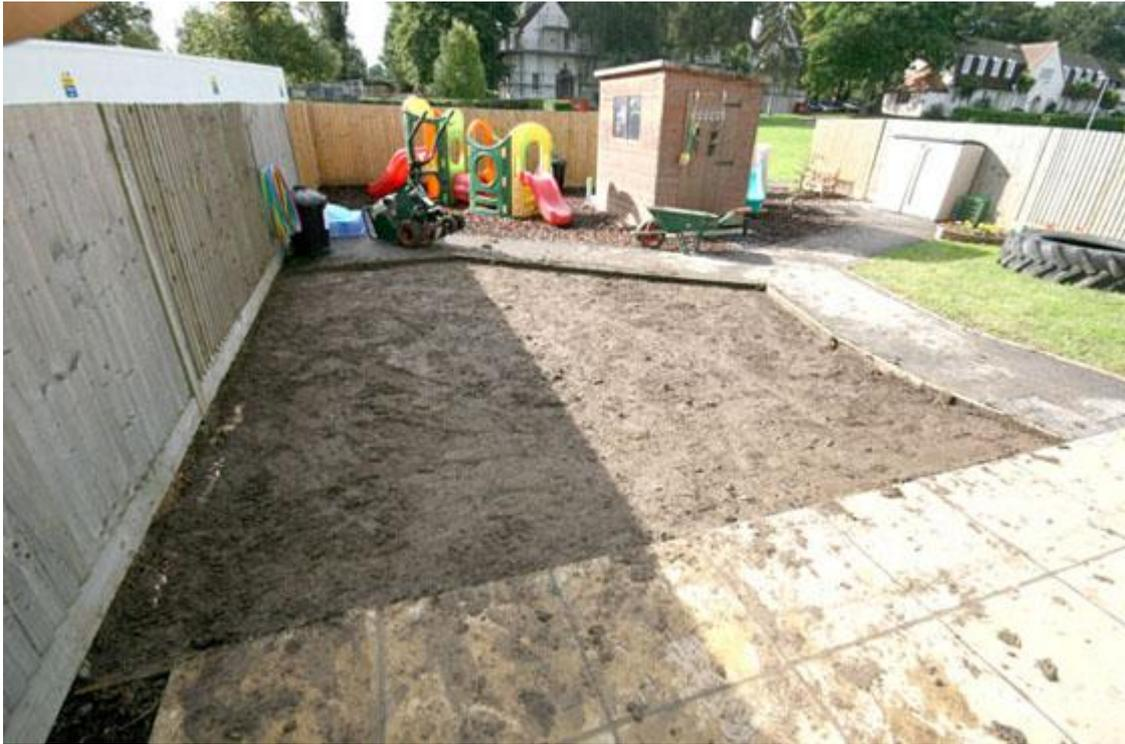
**With all turf removed, the area is ready for the sub base to be installed. As you can see from this image, there is a firm edge all the way around. If installing up to a flower bed, tanalised timber edging or metal edging should be installed.**
