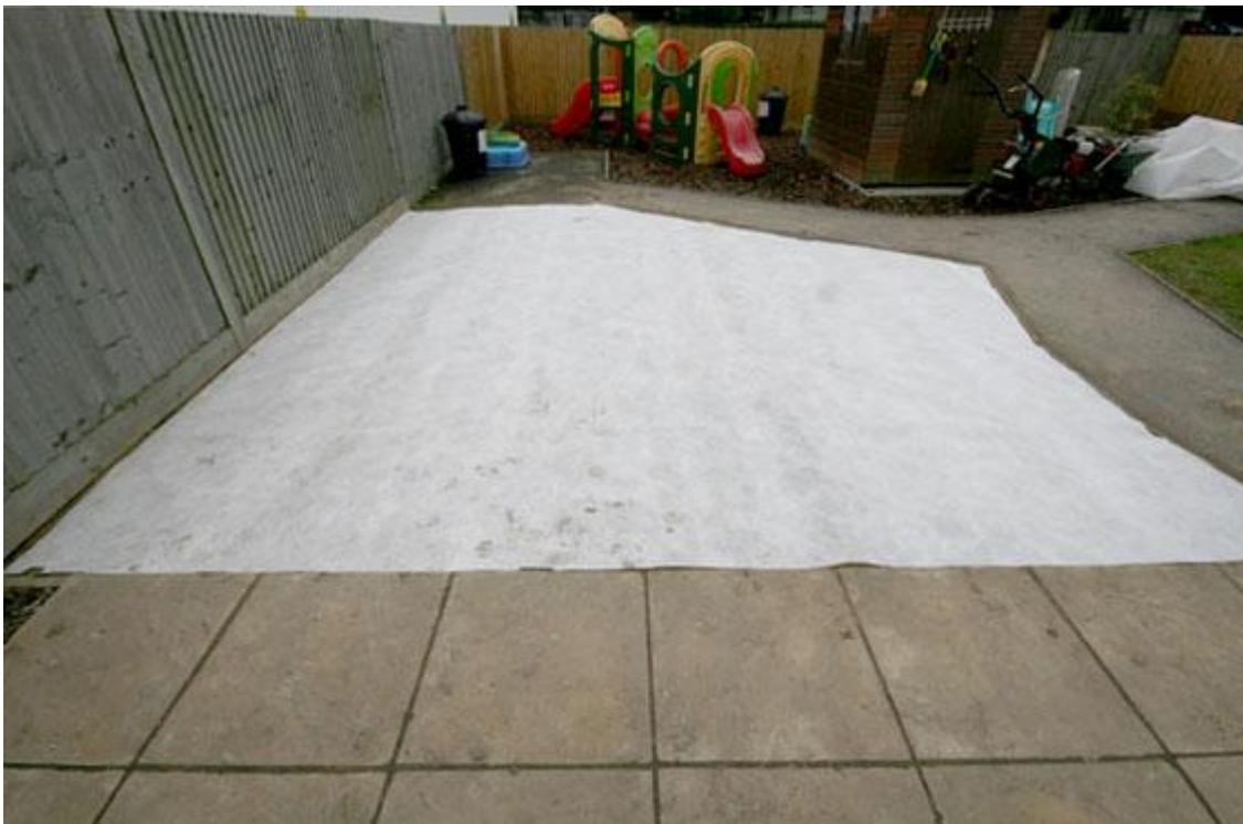
**Install the second layer of geotextile weed membrane and pin in position with 6 inch**
